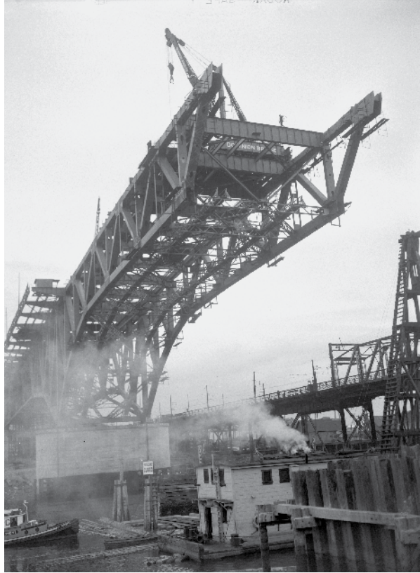
Early construction on the new Granville Street Bridge, Vancouver; 1950s.
